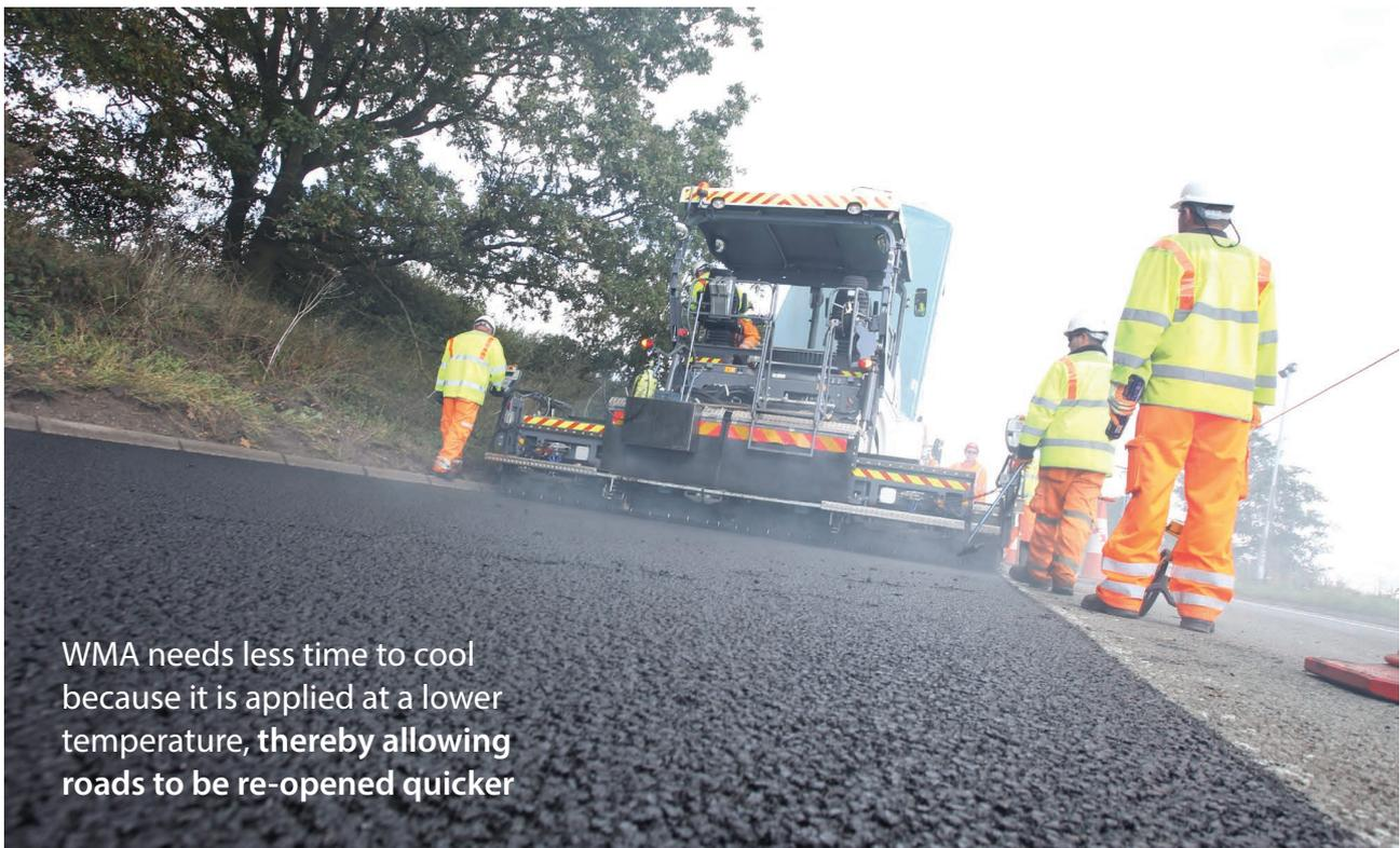
WMA needs less time to cool because it is applied at a lower temperature, **thereby allowing roads to be re-opened quicker**
